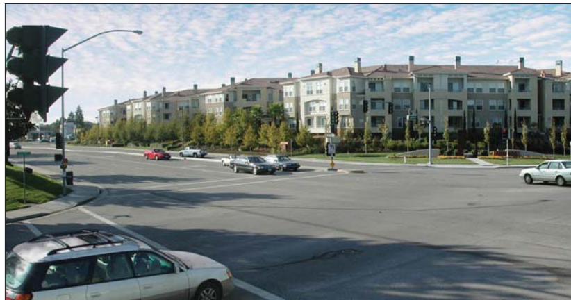
A residential complex in an environment automobile dominated area.
