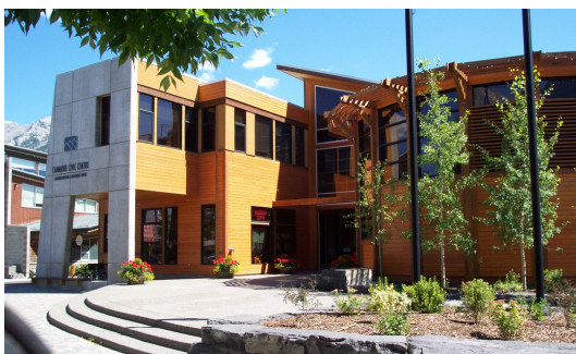
The Town of Canmore's new Civic Centre
